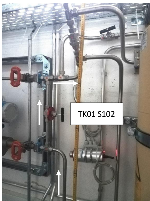
Figure 9 : Piping at compressor bypass
