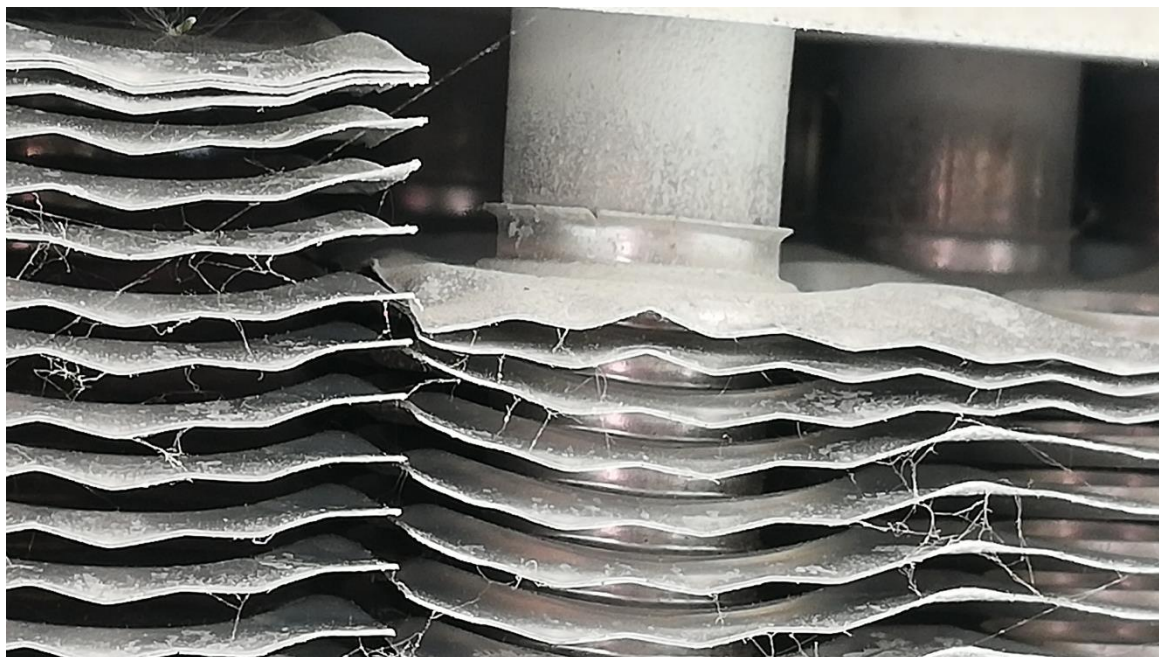
Figure 5 : Pipes and fins inside the UHS
